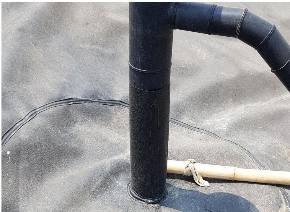
Figure 22 Contouring work for preparation of capture of LFG from existing landfill (Semarang, Java).
