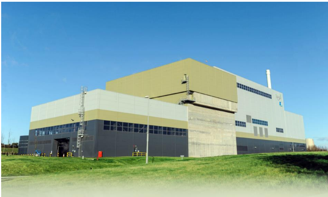
Figure 12. Indaver. Ireland's first WtE plant. Delivers electricity to 20,000 households through the city's grid. Capacity to process approximately 200,000 tons of waste per year 20 .
