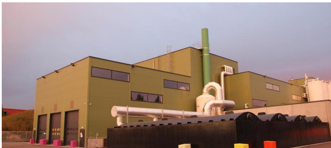
Figure 35. Biogas plant for replacing LPG for busses in Oslo, Norway.
