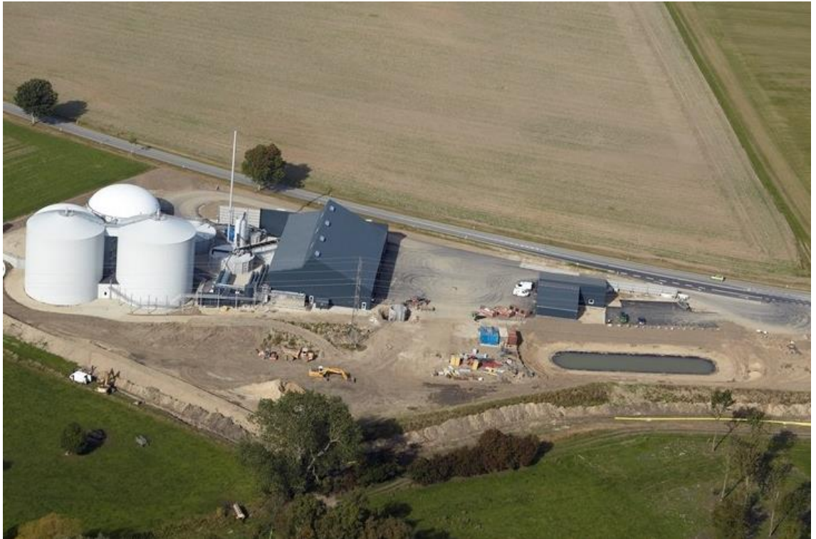
Figure 32. Biogas plant in Solrød Strand Denmark.
