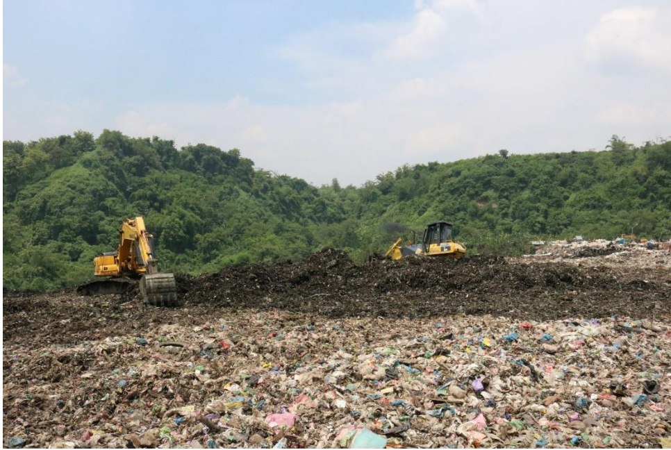
Figure 22 Contouring work for preparation of capture of LFG from existing landfill (Semarang, Java).
