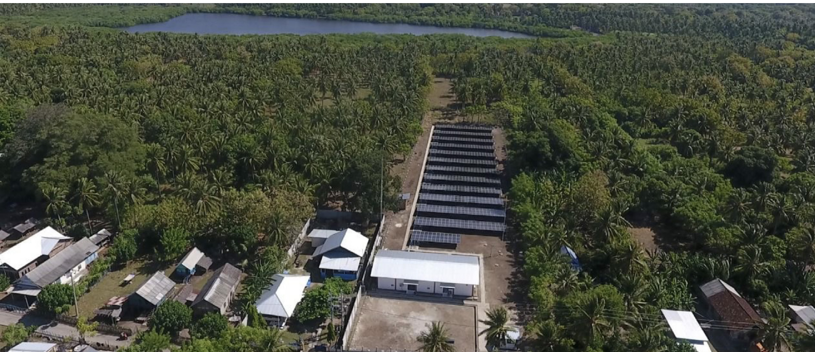
Figure 2. The Solar PV Power Plant on Medang Island, Sumbawa, WNT, has a capacity of 314 kWp and is equipped with a 550 kWh battery and an inverter, supplying 2,574 households on the 4.35 km 2 island with 24-hour electricity (Photo source: PLN)
